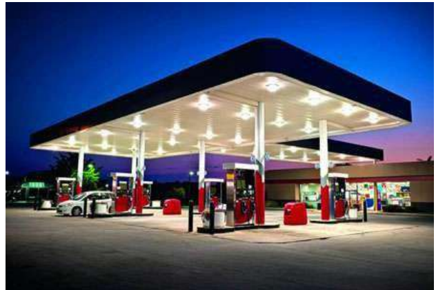
OIL FILLINGS/CHANGING STATION
